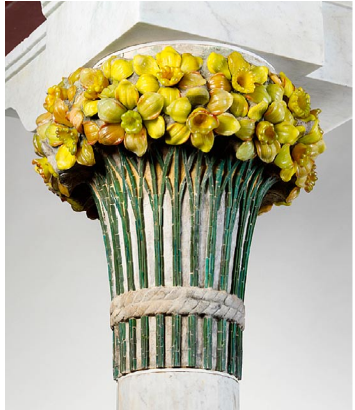
The Daffodil Terrace was named after lovely floral column capitals, featuring daffodils in embedded cast and cut glass, in precast natural gray concrete.
