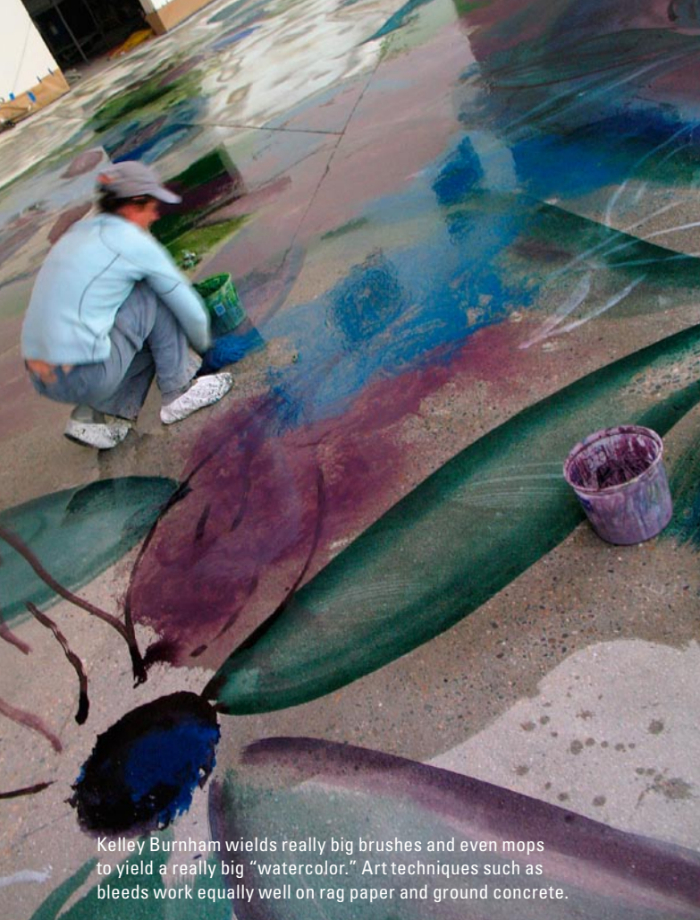
Dye and pigment washes allow nuances of the ground concrete substrate, such as aggregate cross sections and craze cracking, to show through. In California, these are called “bitchin’ details.”
