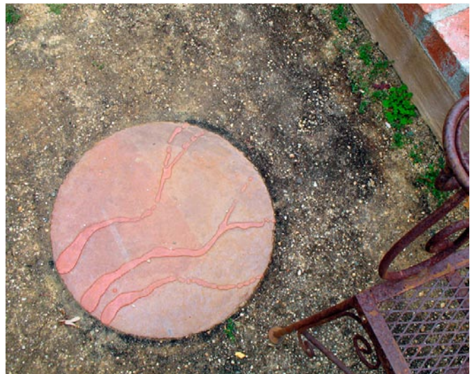
Martin Webb stained over troweled integrally colored skins (overlays) on these mixed-media horizontal and vertical artistic architectural elements.
