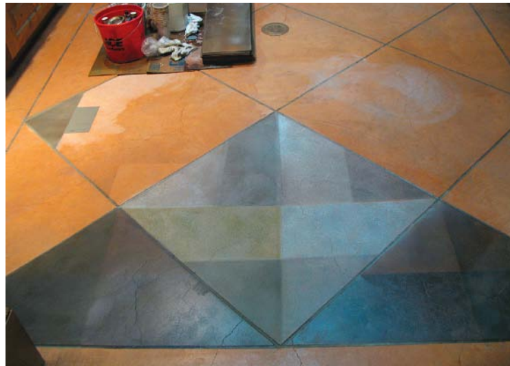
To define “that special gray” for Restoration Hardware in San Francisco, mock-ups at the site explored grinding, staining, dyeing, tinting and sealing.
